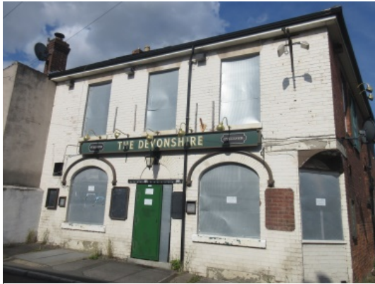
Principle (west) elevation of the site, taken from Occupation Road
