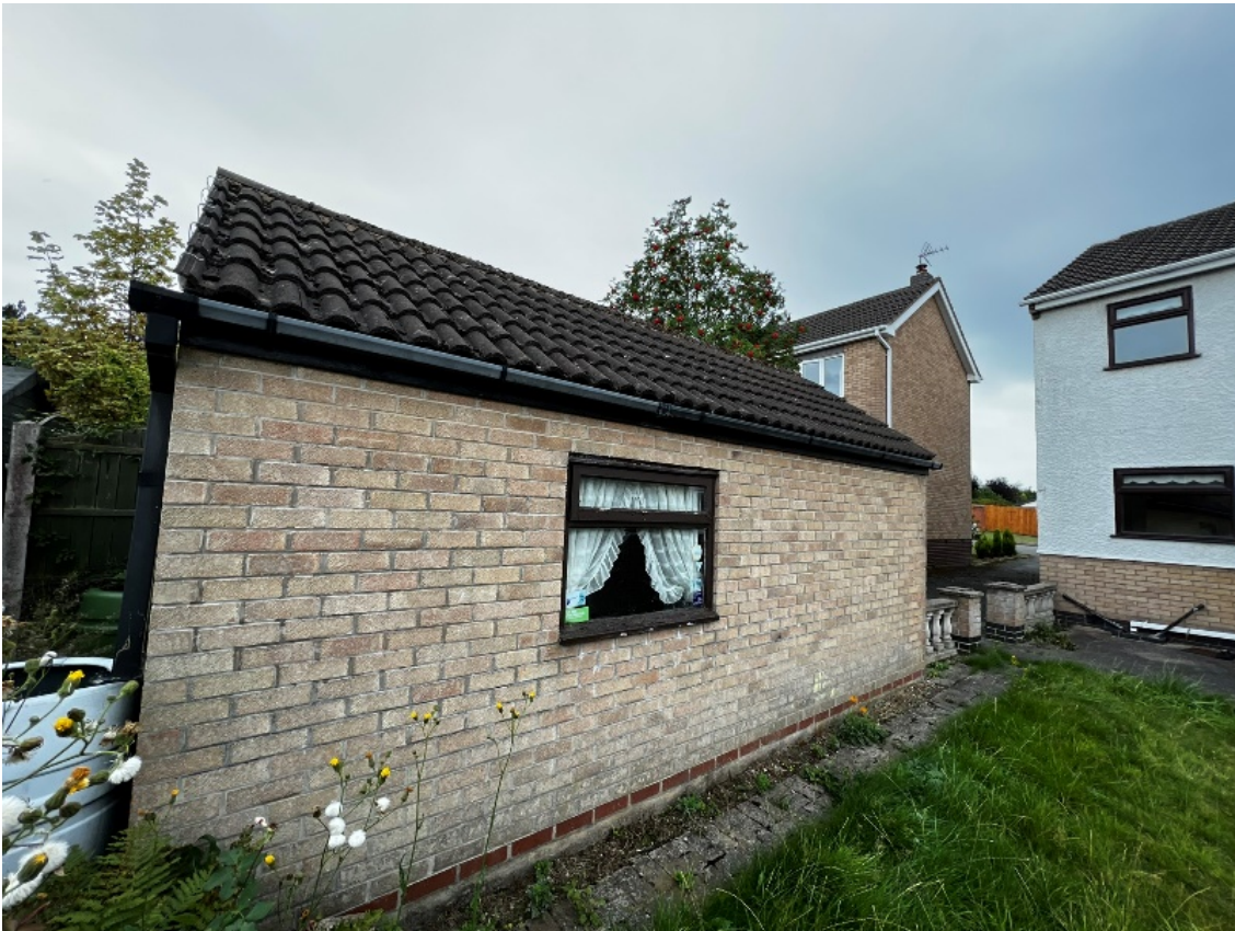
Figure 6 - side view of the site detached garage from the rear garden
